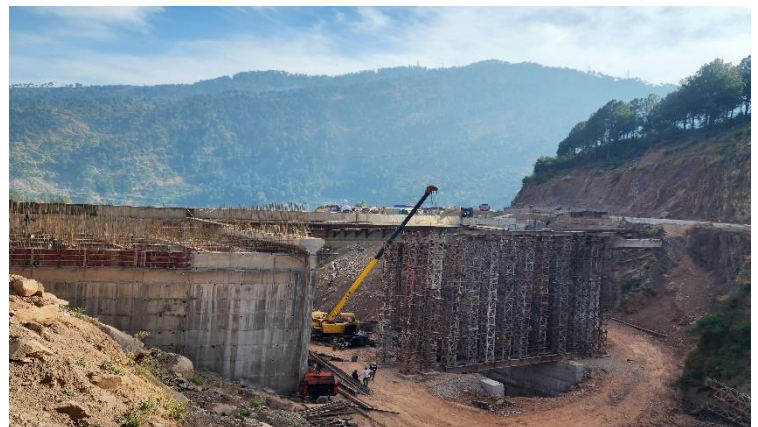
MNB 32- Spill Through Abutment
