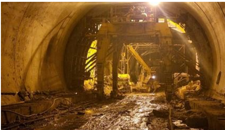
Chandrakot Tunnel Udhampur Ramban Project
