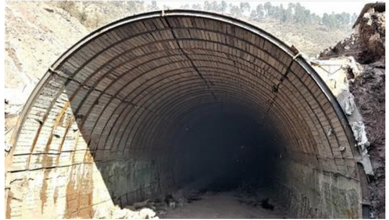
Tunnel Cut and Cover Under Construction
